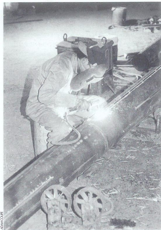
A welder at work in the Nepal Hydro & Electric workshop.
